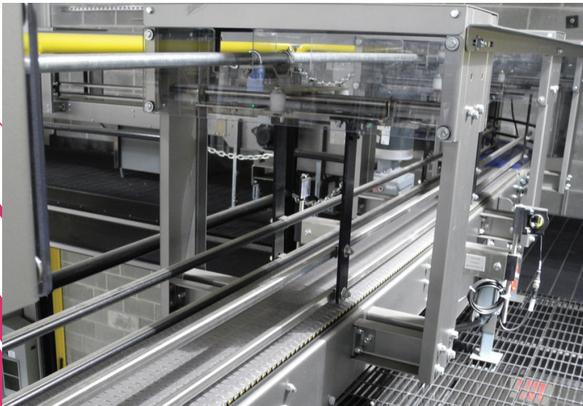
Dual lane system utilizing electric actuated cylinders.
